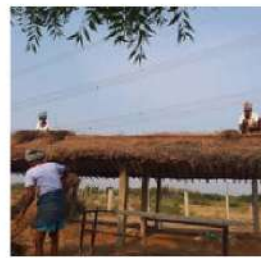
Securing the ridge with split bamboo
