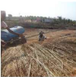
Holding the first layer by split bamboo
