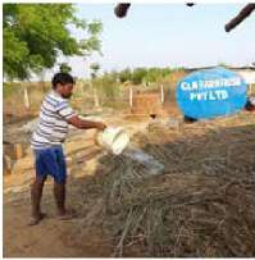
Piling bunches and soaking them in water a day prior to laying
