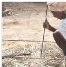
Typing bamboo through thatch with the giant needle & wire
