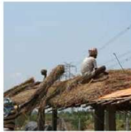
Collecting bunches and spreading for first layer
