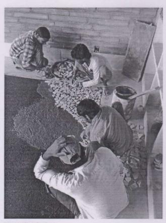
Source: Case Design Mosaic paving is formed from waste stone pieces from quarries in Rajasthan and Gujarat
