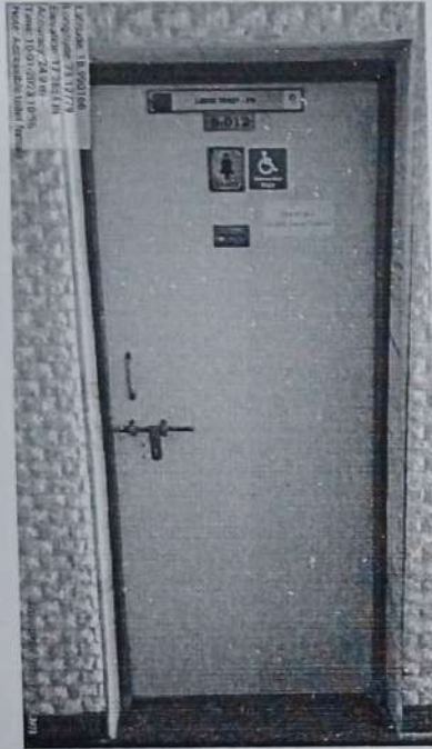
Ladies toilet for Differently abled
