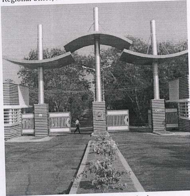
Entrance Gate, ARCI, Balapur, Hyderabad
