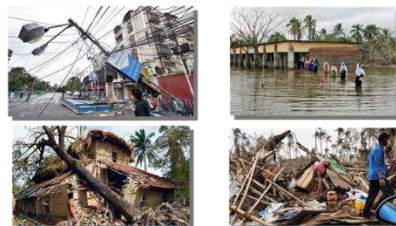
The loss in terms of architecture due to Cyclone Amphan was substantial. The cyclone caused extensive damage to buildings, infrastructure, and architectural structures in the affected areas. Many homes, schools, hospitals, and other buildings were destroyed or severely damaged by the strong winds and storm surges brought by the cyclone
